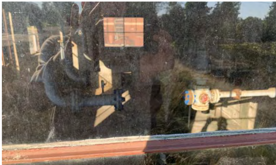
Interior of gas house
