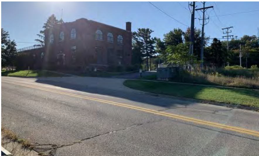
Property adjacent south, facing south
