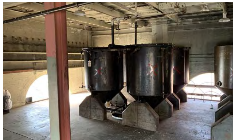
Empty heavy oil tanks on third floor mezzanine
