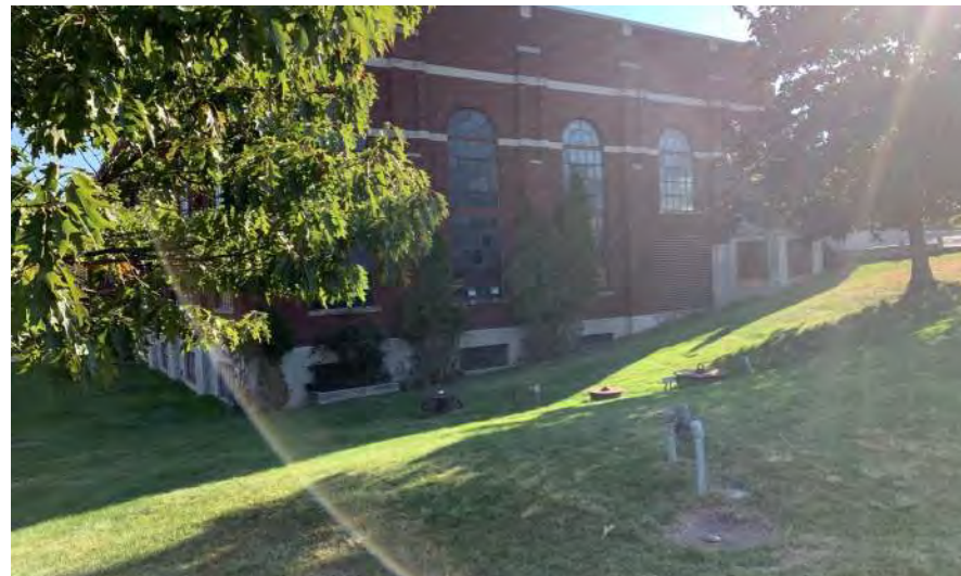
West side of building facing northeast
