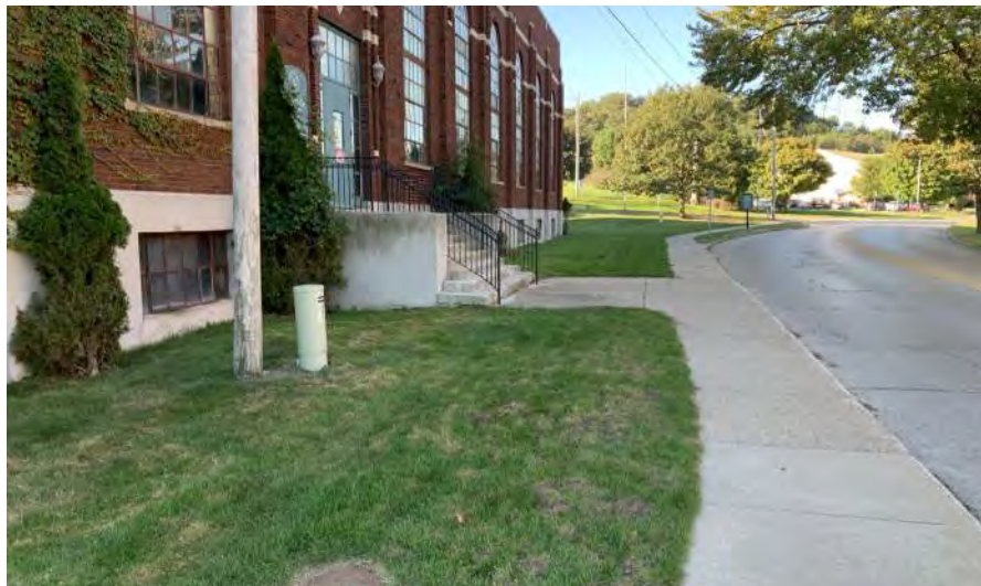
North side of building facing west
