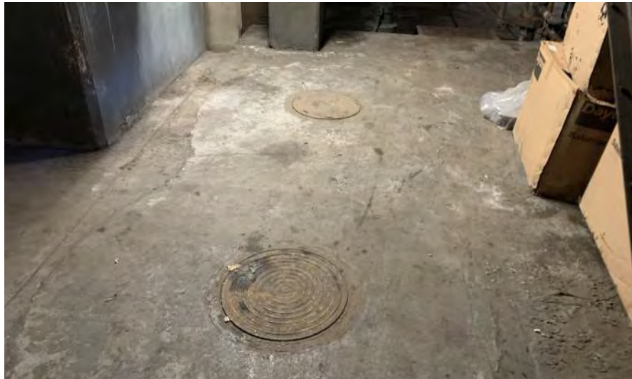
Manhole covers in basement
