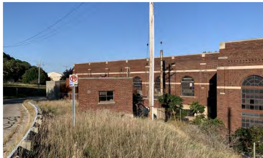
Site building facing northwest with gas house in foreground
