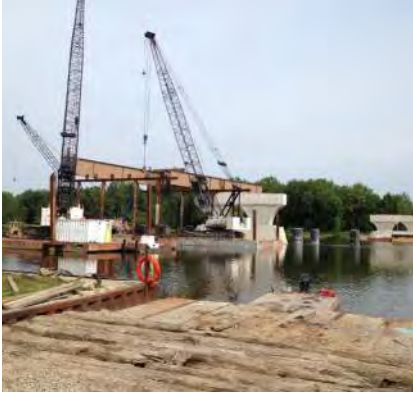
US 31 Bypass, under construction
