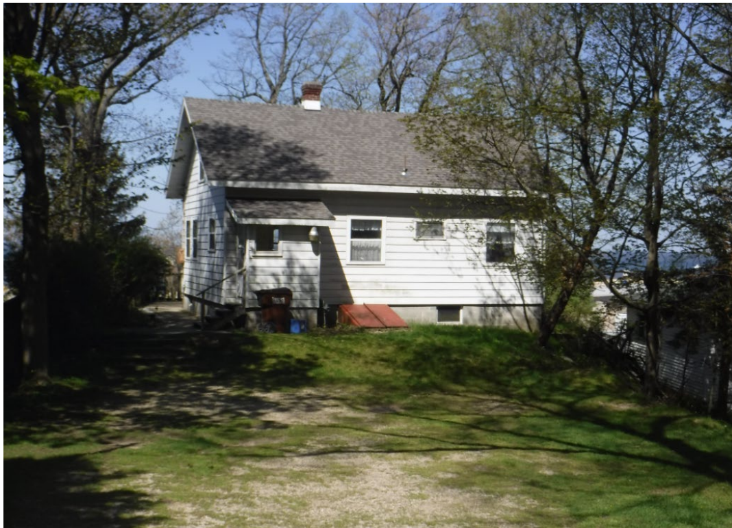
Existing home (rear view)
