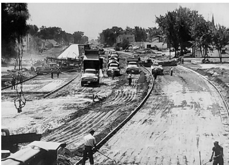
The old US-31 was re-routed in the 1950s, becoming a divided highway with four lanes (instead of two), and was known thereafter as Beacon Boulevard. (Credits: Sawyer, 2025.)
