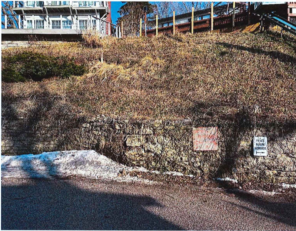
Overall view of retaining wall and slope above.
